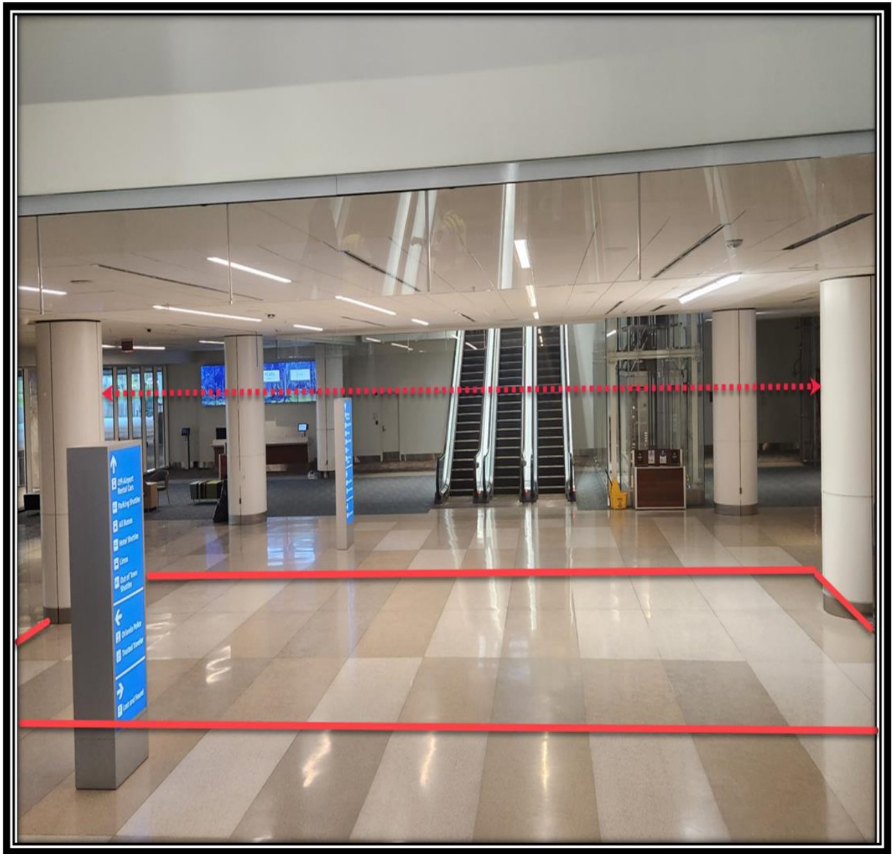
Approved location is the tiled area between the two (2) columns.
